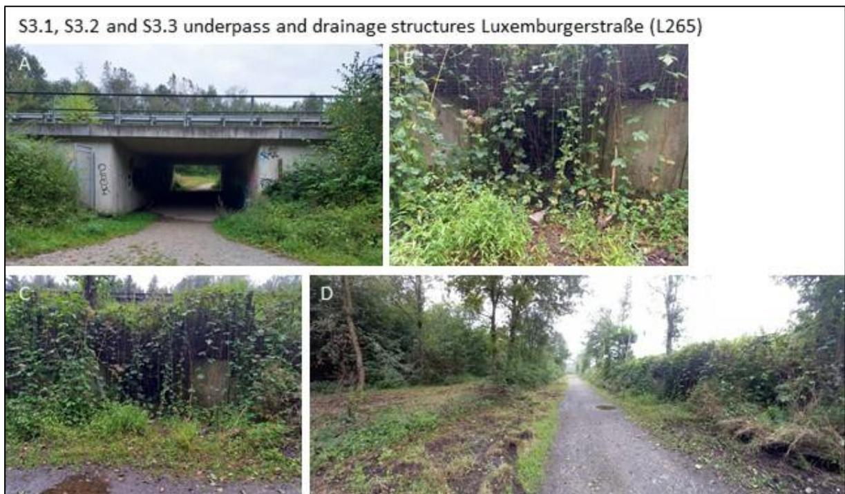
Figure 36: S3.1, S3.2 and S3.3 underpass and drainage structures Luxemburgerstraße (L265). **A:** S3.1 underpass L265. **B:** S3.2 drainage structure with sheep wire fence **C:** S3.3 drainage structure with sheep wire fence. **D:** vegetated sheep wire fence along north side of L265.
